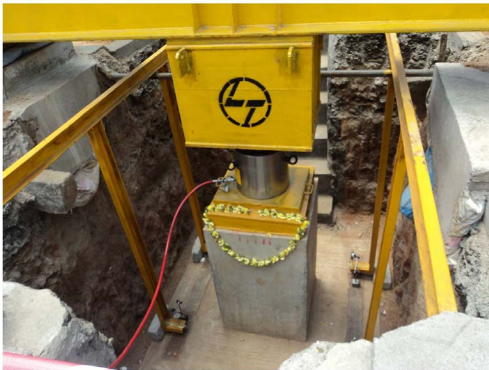
Load Test in progress
