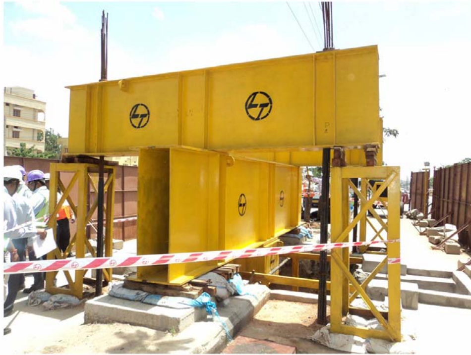
Load Test in progress
